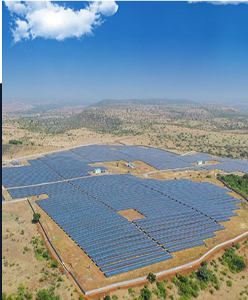
100MW + Capacity installed in Ground mounted
